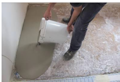
Application of PLAN LEVEL 315
