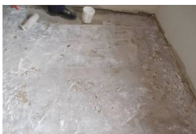
Application of MICROART AD 21 primer
