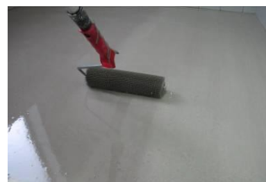
Levelling of the surface with a spike roller
