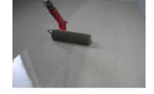
Levelling of the surface with a spike roller
