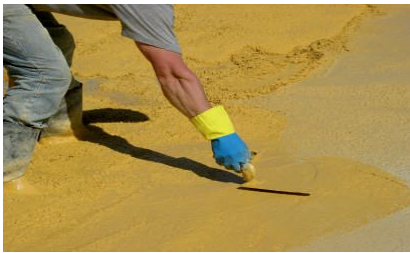
1. Trowelling of SCALA DECOR's fresh surfaces
