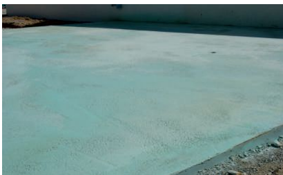
3. Waiting time until the bottom layer hardens
