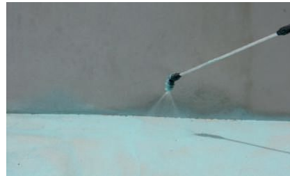
2. Spraying of SCALA AD 32 on fresh surfaces
