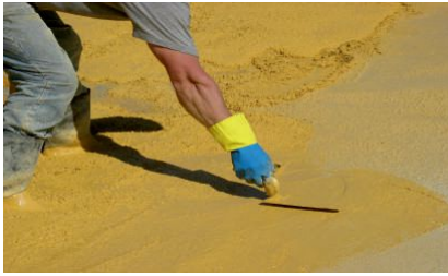
1. Trowelling of SCALA DECOR's fresh surfaces
