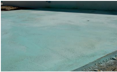
3. Waiting time until the bottom layer hardens
