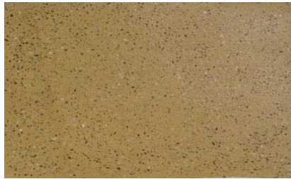
5. After curing is complete, application of surface protector B-REPARA PROTEÇÃO AD40
