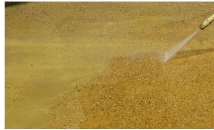
4. Removal of the surface layer by water jet, exposing the aggregate
