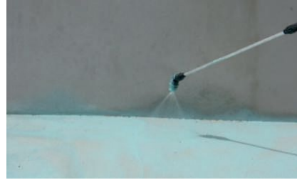
2. Spraying of SCALA AD 31 on fresh surfaces
